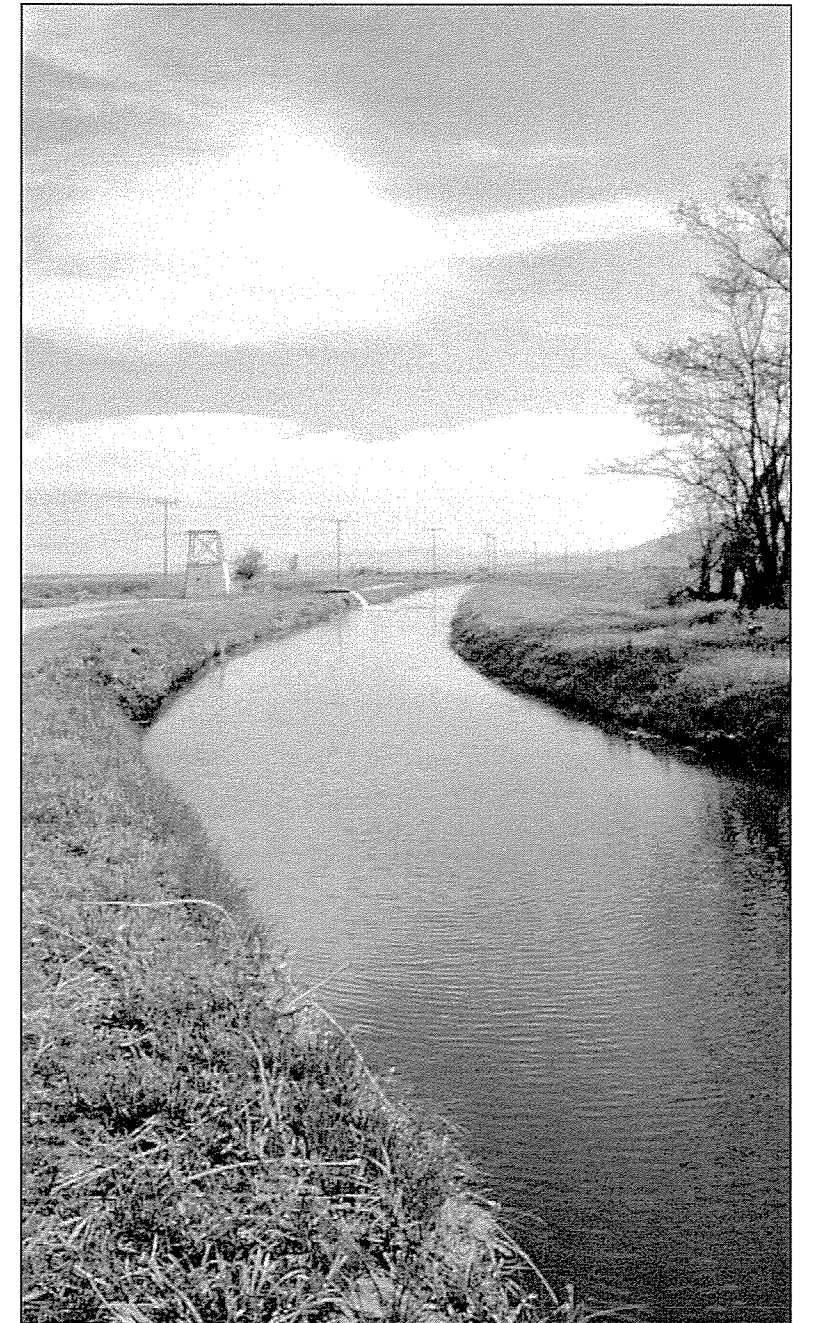
The upper and lower McNally canals in the Laws area are LADWP conveyances used to supply water from the Owens River to LADWP irrigated leases and spreading facilities. These canals are the primary source of recharge to the Laws area. LADWP also uses the canals to convey groundwater pumped from the Laws wellfield to the river for export to Los Angeles.
