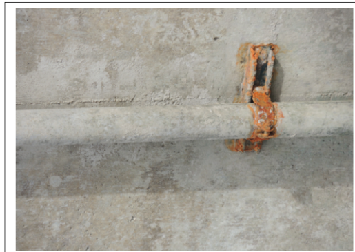
The communication pipe is A304 stainless steel, but the Uni-strut wall straps were only galvanized steel. All three wall brackets need to be replaced with A316 Stainless steel uni-strut and bolting.
