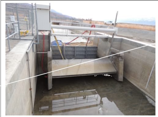
View of the cleaned and pressure-washed Langemann Gate ready for inspection . Note the downstream bulkhead gate and the dirt coffer dam preventing the river from flowing back into the sand trap.
