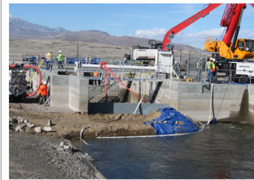
View from rail car bridge at the downstream coffer dam. The lower 225 LF of tailrace channel below the LG is filled 3 to 4 Ft. deep with sands and river sediments. This needs to be cleaned also.
