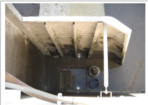
Top view of a LG side plate with stand-off bar. Although the LG was constructed of A304 stainless steel, the thin side plate metals were only plated stainless steel which corroded at seams & welds.
