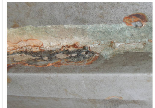
Typical rust-through holes in both of the original gate side plates. A quote of $ 9,900 dollars was received in 2016 for new side plates constructed of A316 corrosion-resistant Stainless Steel.
