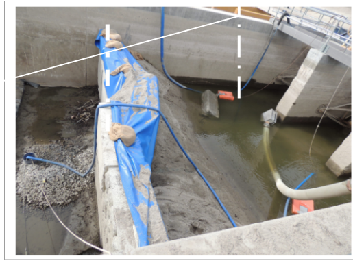
Crews installed concrete barrier blocks and tarp D/S of the three radial gates to prevent inflows from the 3 leaking radial gates tarped, but never sealed.
