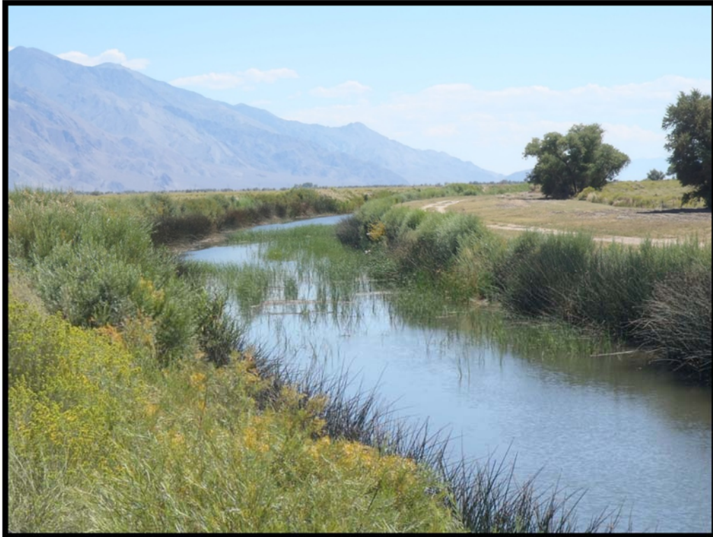
Figure 2-26. Inset marsh occluding LA Aqueduct in response to reduced flow.
