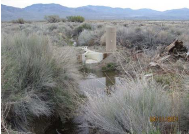
Warren Lake Project, April 2011 New Parshall Flume, Flow Meter Installed
