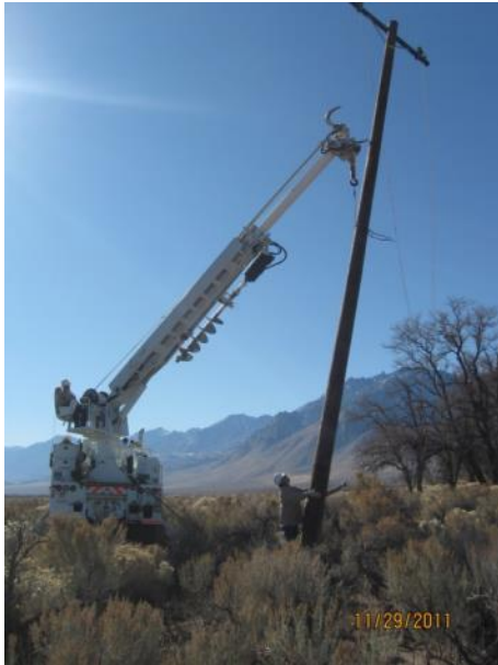
Hines Spring Well 355, November 2011 LADWP Erecting Powerline to Power Well 355
