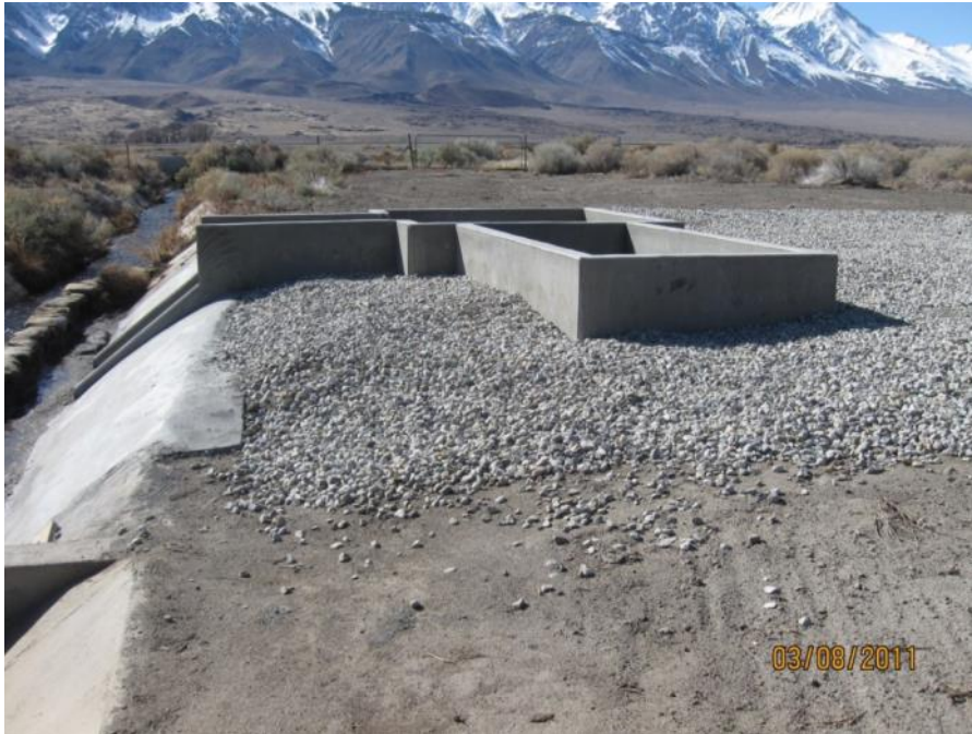
Aberdeen Ditch Project, March 2011 Concrete Diversion Structure With Fish Barrier
