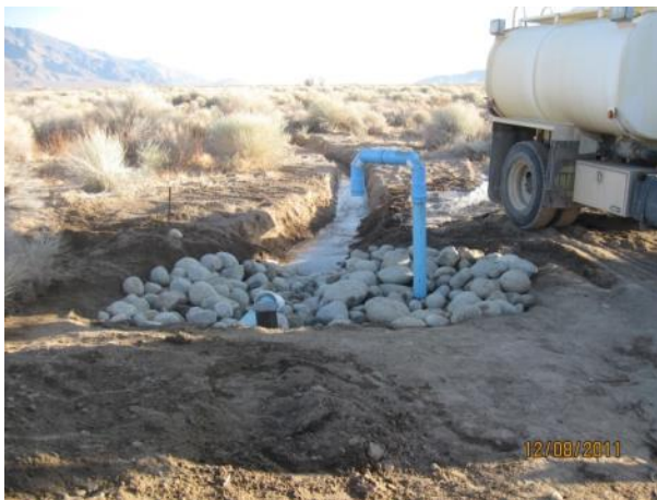
North of Mazourka Canyon Road Project, December 2011 Pipe Outfall (convergence of both pipelines) Within Exclosure During Implementation
