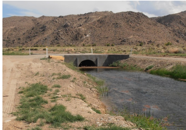
Big Pine Canal/Warren Lake Project, July 2014 New Check Wall and Road Crossing
