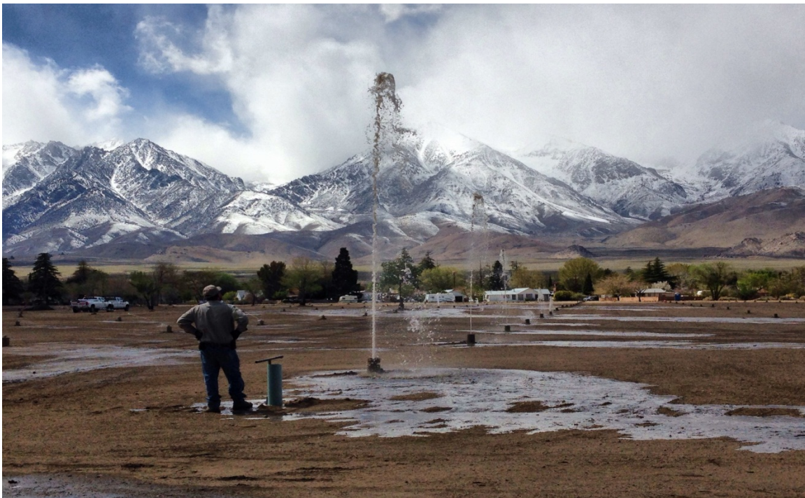
Figure 6.5. LADWP worker clearing the newly installed irrigation line at the Independence Eastside Regreening project.
